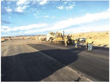
**BULLHEAD CITY** — It's a race against time at Laughlin/Bullhead International Airport as they have a two-week window to pave the runway and parallel taxiway, both of which are being extended 1,000 feet for a total length of 8,500 feet. The airport is closed to all aircraft except helicopters until Dec. 21, said Jeremy Keating, airport director.
